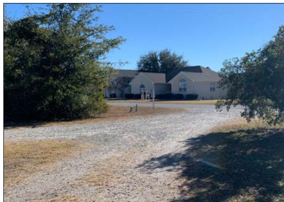
Existing conditions looking south to Settlers Lane
