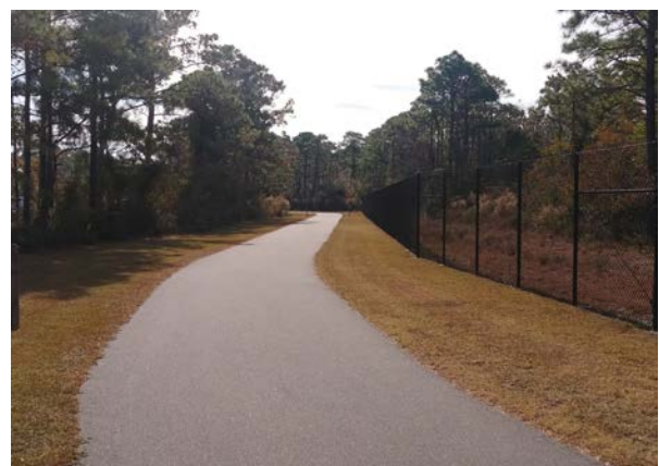
Photo: the Island Greenway in Carolina Beach. A potential project proposed in this Plan would extend the greenway on MOTSU land, offering greater connectivity for Kure Beach residents.
