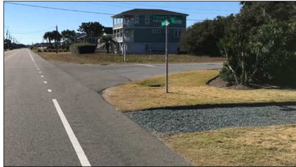
Existing conditions along Fort Fisher Blvd.
