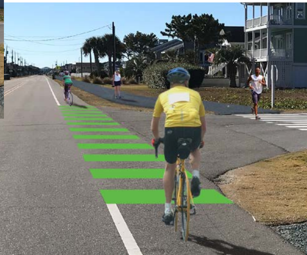
Example of high visibility bicycle lane intersection markings.
