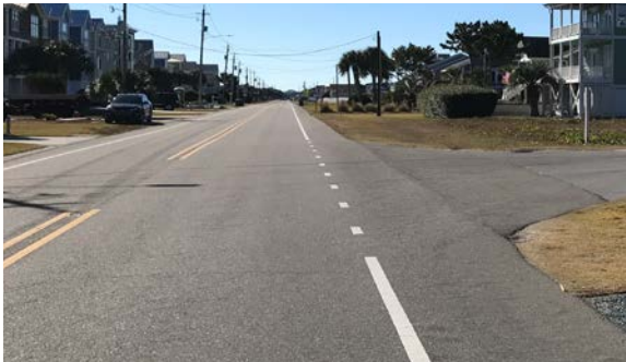
Existing bicycle lanes on Fort Fisher Blvd with 4 inch white dash intersection markings.
