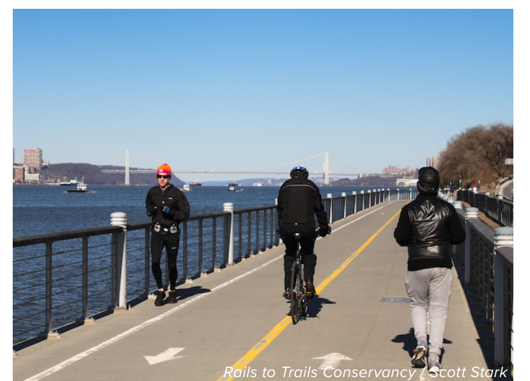
SUFFICIENT TRAIL WIDTH (>10 ft) reduces conflicts when passing, and allows faster traffic to pass slower traffic.
