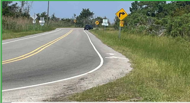
28 Existing Bike Lane on Fort Fisher Blvd
