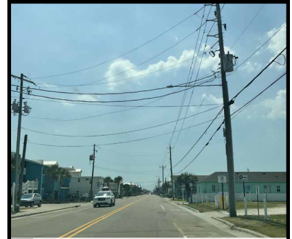
24 Utilities on Fort Fisher Blvd
