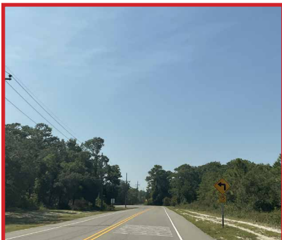
17 Ditch on West Side of Dow Rd
