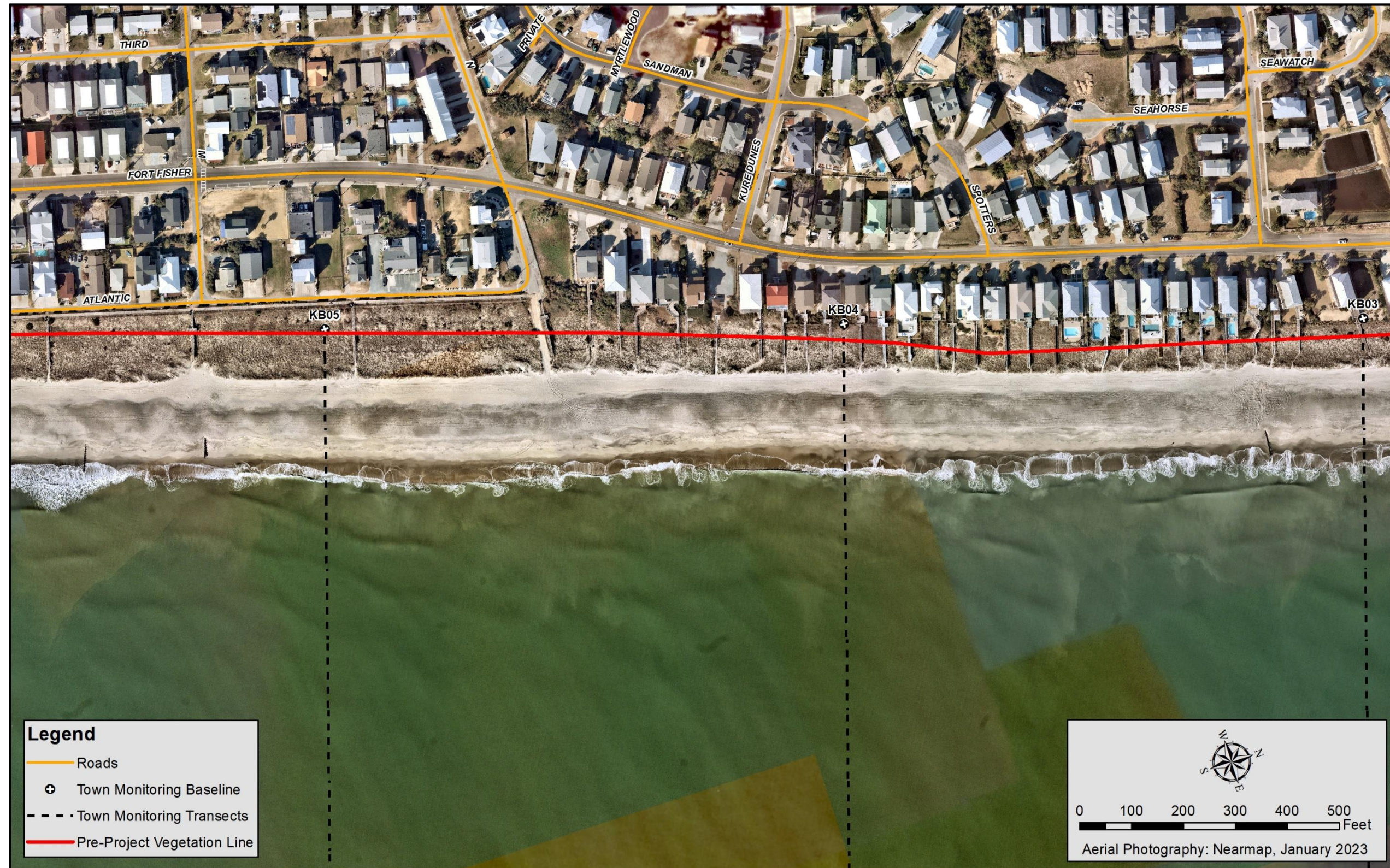
Figure 3-2. Kure Beach Pre-Project Vegetation Line (2 of 6)
