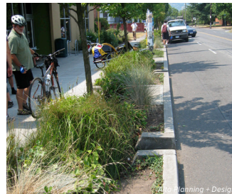
GREEN INFRASTRUCTURE such as bioswales, bioretention planters, rain gardens, and permeable pavements can help manage stormwater.
