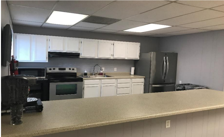
Community Center kitchen sink
